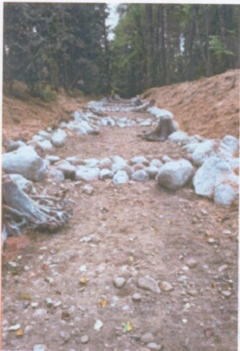
Pictured above: Newbury weir created in stream restoration in Coquitlam
